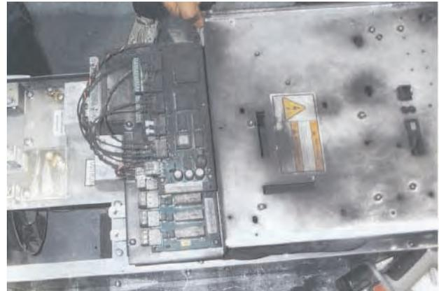
Photo 1, Fan Injecting Dust into Drive Enclosure
