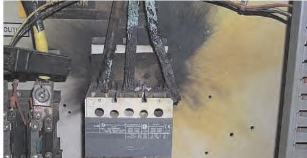
Photo 3, Arcing Caused by Loose Input Contacts
